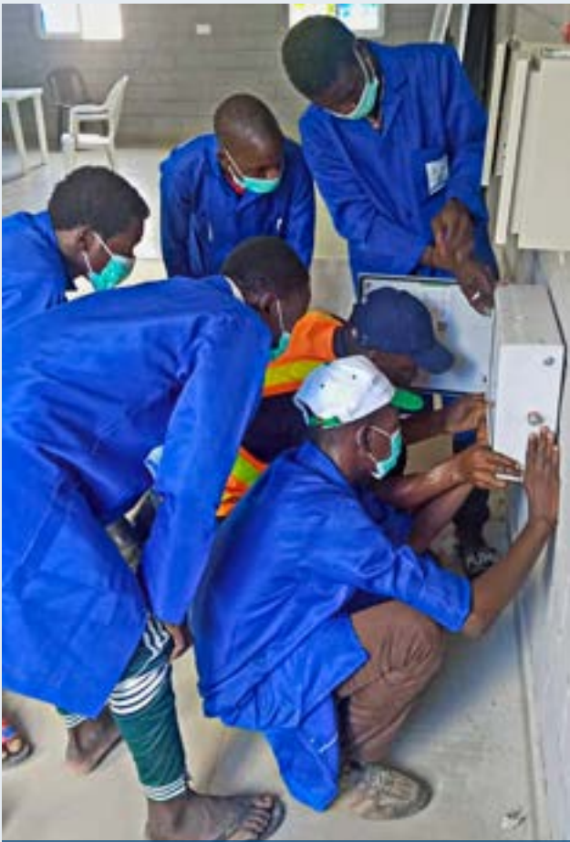
Solar PV installation and maintenance
