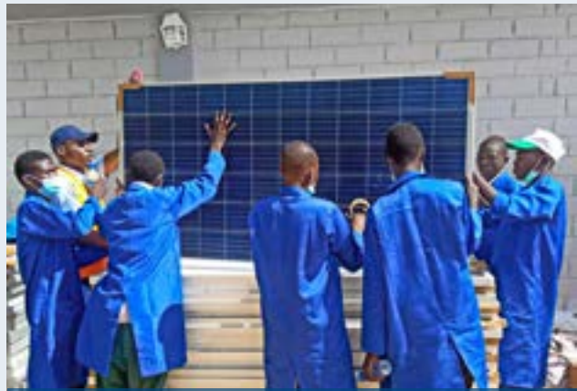
Solar PV installation and maintenance
